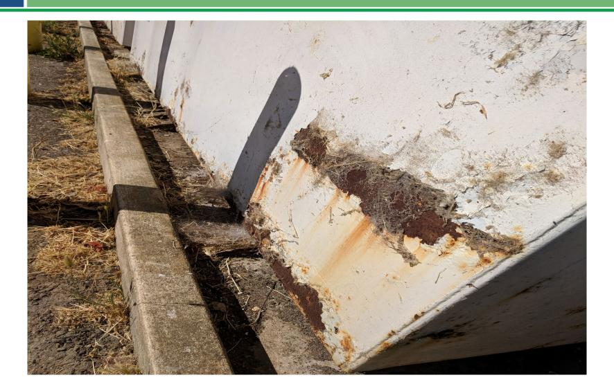
Fuel tank at a marina facility with visible signs of corrosion
