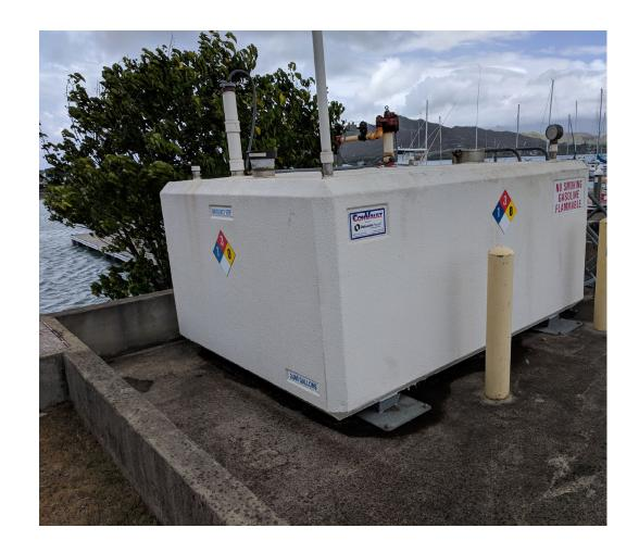
Double-walled marina fuel tank – adequate secondary containment
