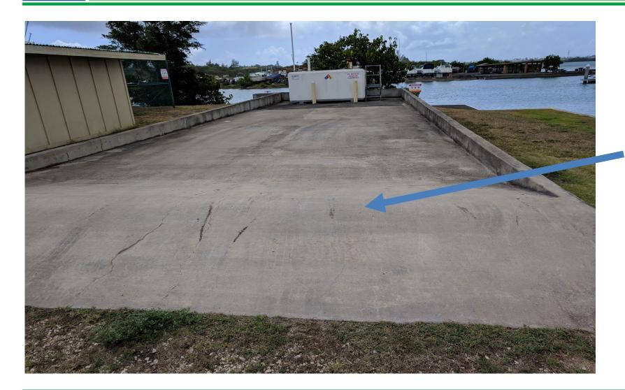
Roll-over berm provides containment for the most likely spill scenario during transfer activities.
